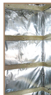
Foil vapor barrier furring strips
