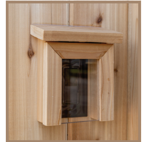
Exterior light switch w/ rain cover
