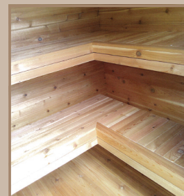
2-Level cedar benches, cedar floor, wall & ceiling
